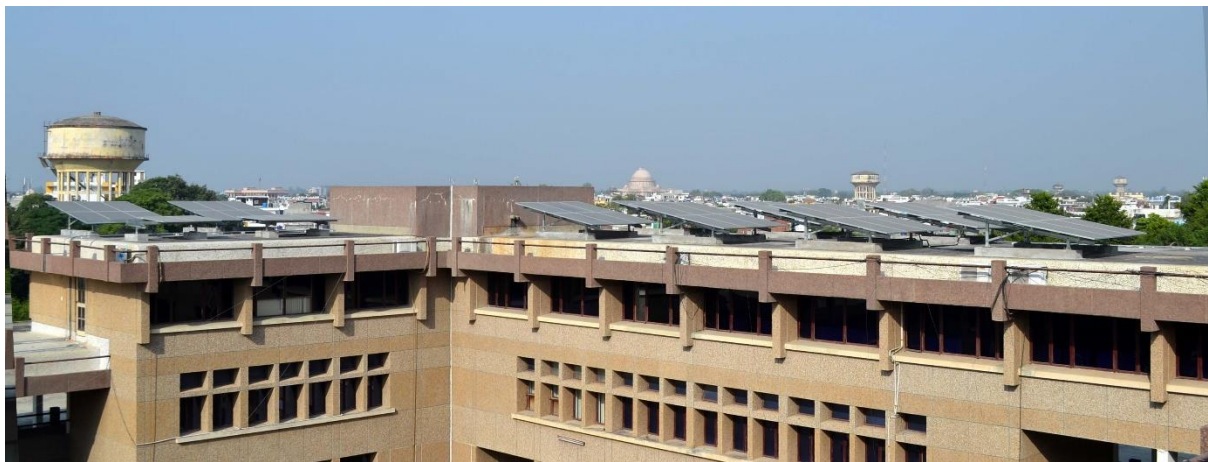
Pic. PV panel in Administrative & Library Building of BIRD
