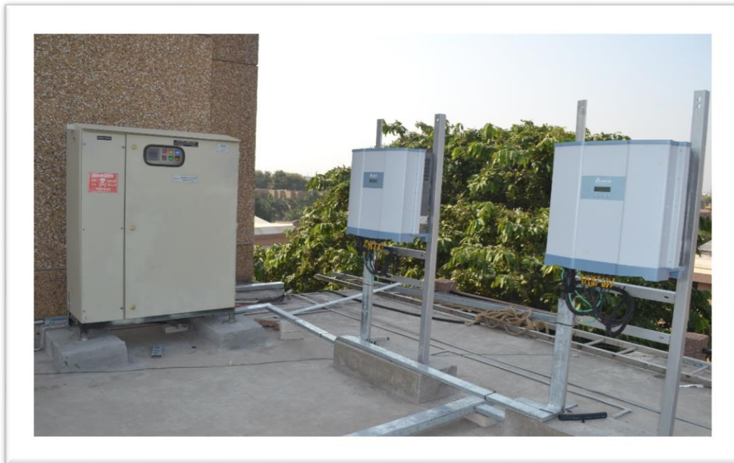
Pic. Control unit of Solar PV System
